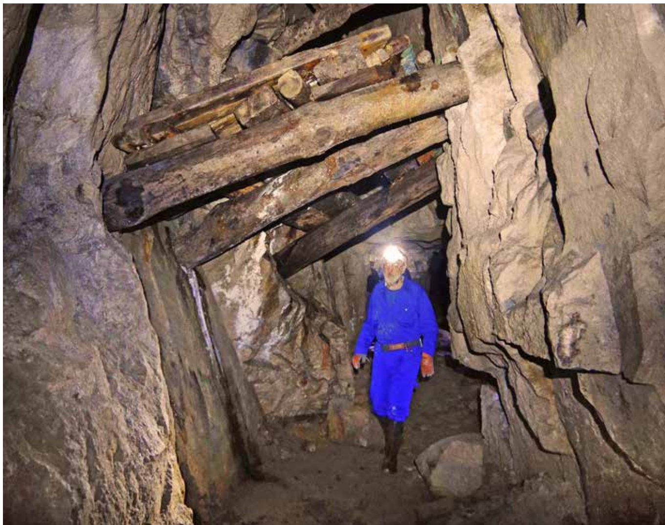
Heavily timbered stope in Cligga mine. Photo Ed Waters
